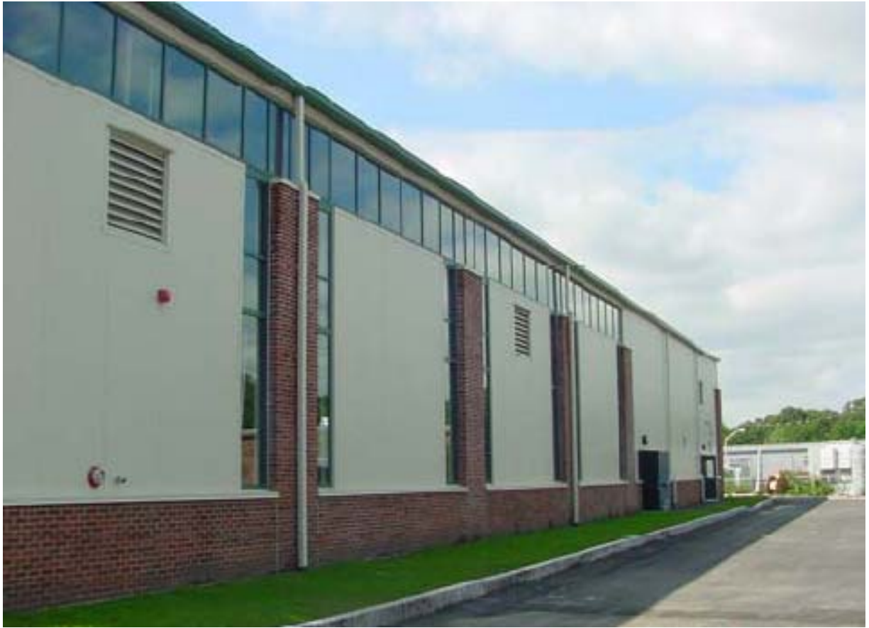
The new Municipal Light Plant garage was recently opened.
